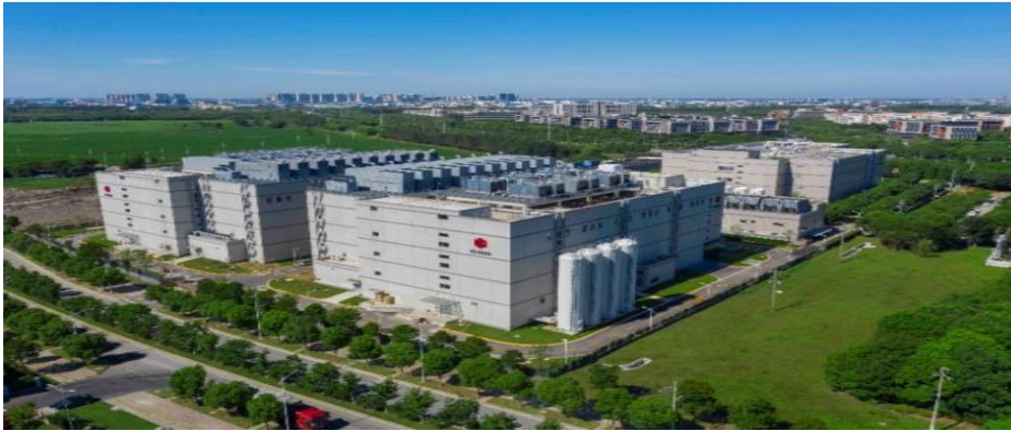
Figure 7. GDS's data center example
